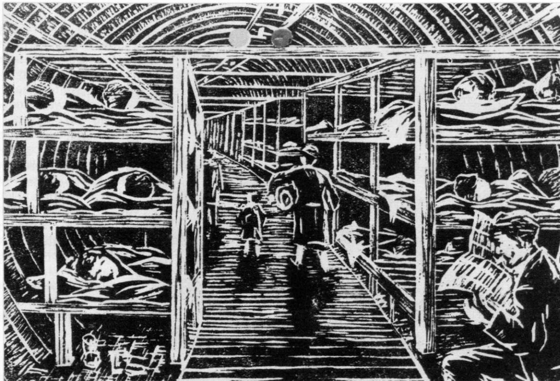
Photographs of the Westdown and Gainsborough shelters have proved impossible to trace but this linocut drawn in 1941 by N.H. Johnson gives a vivid impression of the Gainsborough Bridge Tunnel. The proportions are not quite right for a 12ft diameter running tunnel, however, and the picture gives an impression of space that could never have existed. [Vestry House Museum]
